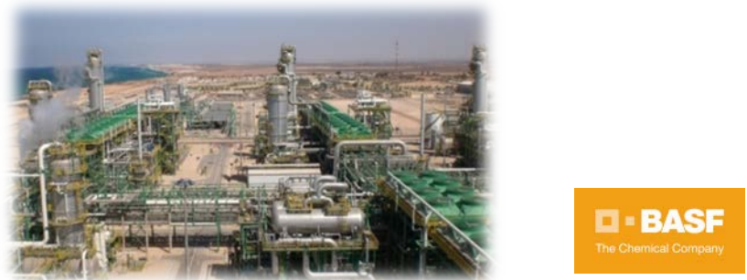
Chemical production complex
