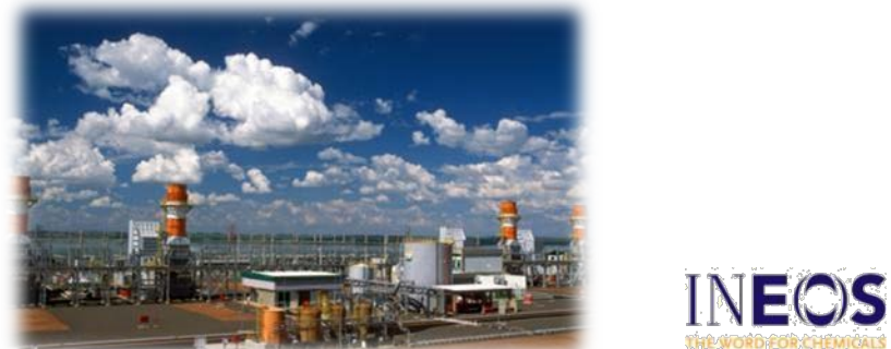
Steam network management of a large interconnected chemical plant
